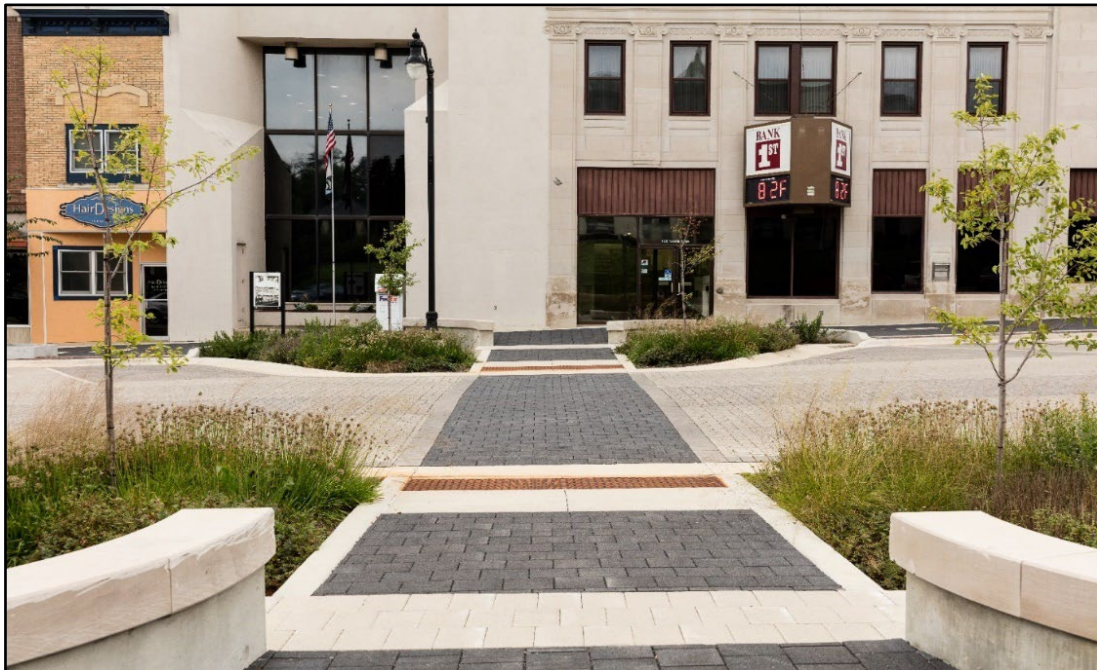
Example of a Mid-Block Crossing West Union, Iowa
