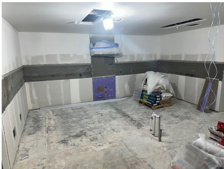
Pictured Above: Future Kitchen
