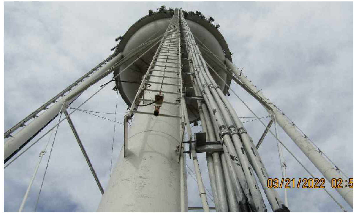
K EXIST. CABLE ROUTE SCALE: NONE
