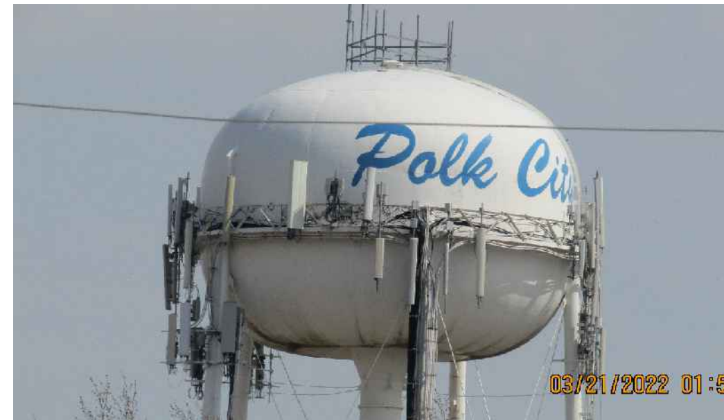
A EXISTING ANTENNA LAYOUT PHOTO SCALE: NONE
