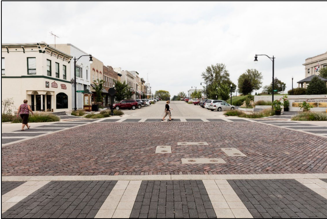
Example of a Raised Intersection (speed table) West Union, IA
